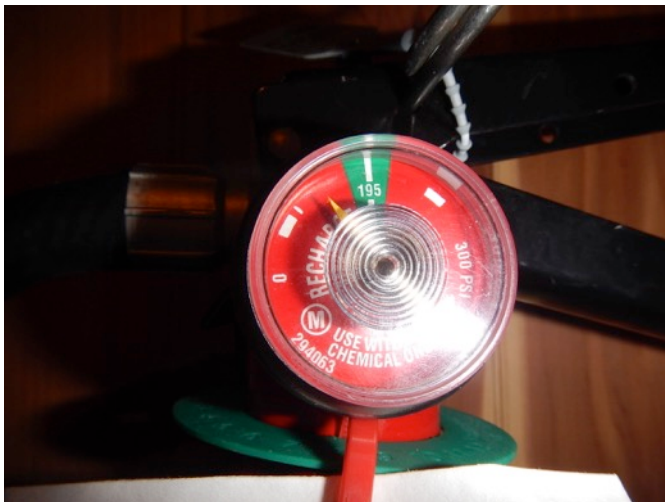
Fire extinguisher charge gauge indicates RECHARGE
