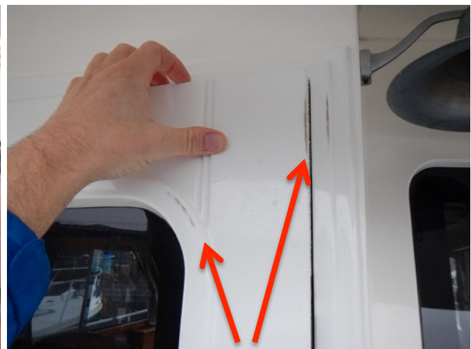
Gelcoat scratching at salon doorframe
