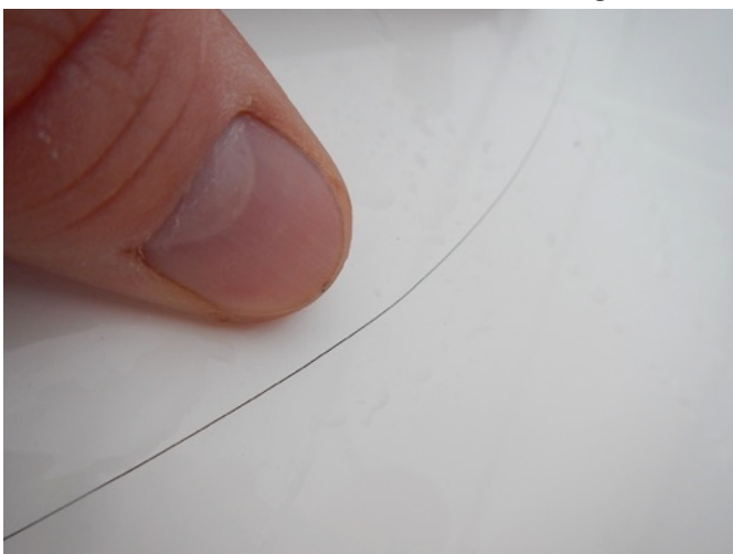
Gelcoat cracking at underside of chain locker deck hatch
