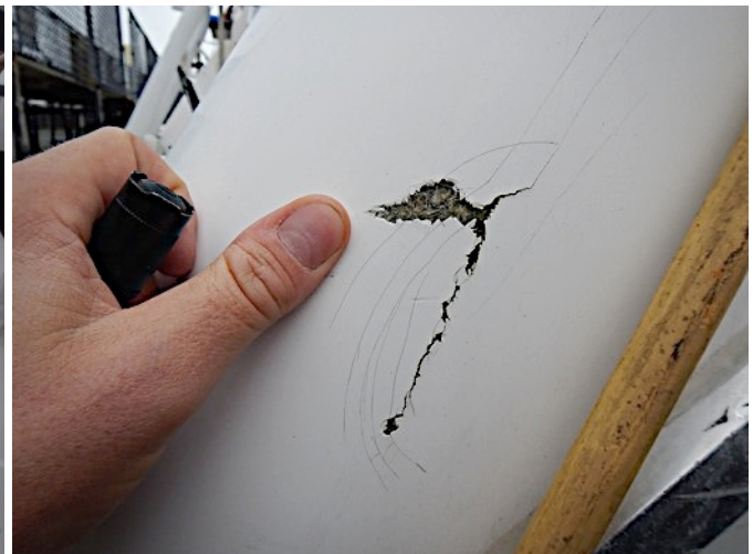
Gelcoat & fiberglass damage
