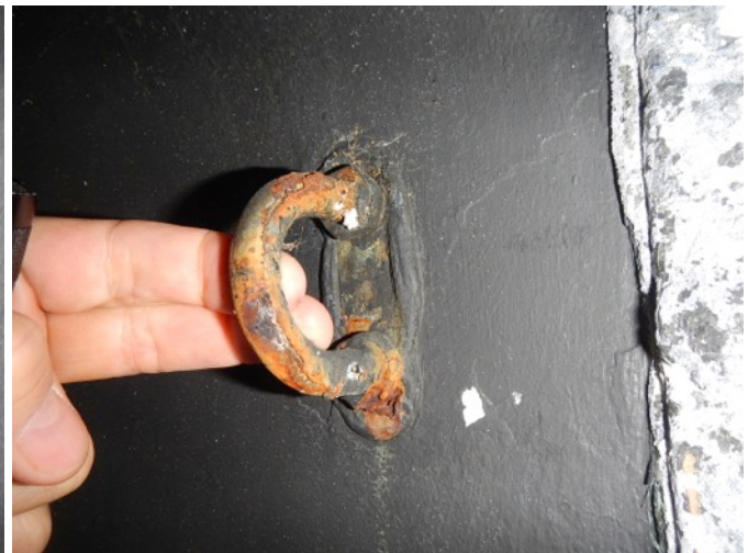
Zinc anodes are deteriorating
