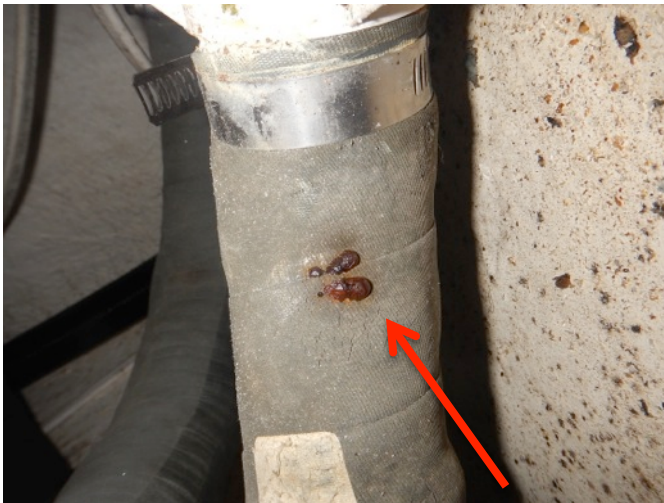
Sanitation system hoses are bulging & leaking
