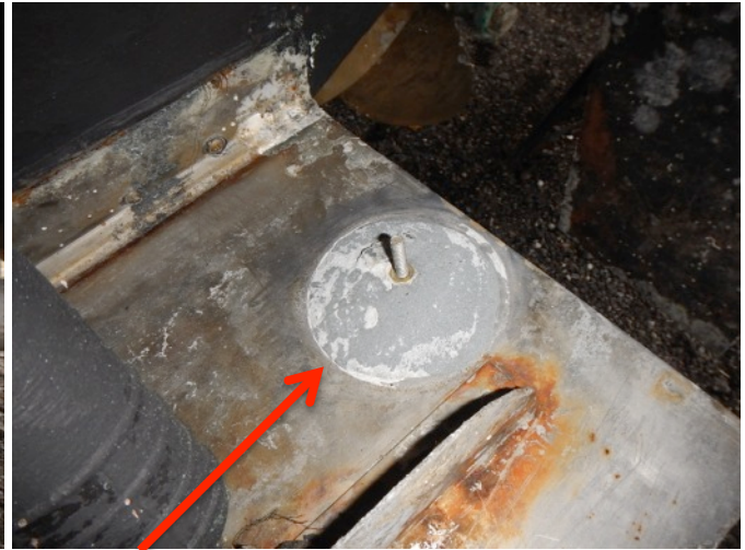
Zinc anodes are deteriorating
