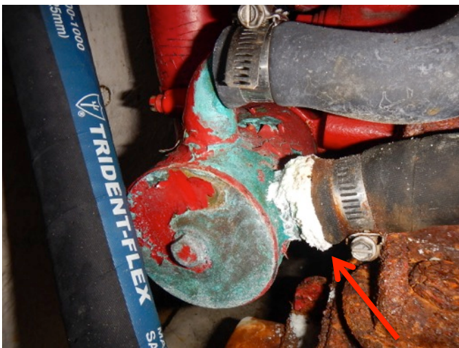
End caps of generator heat exchanger are corroded
