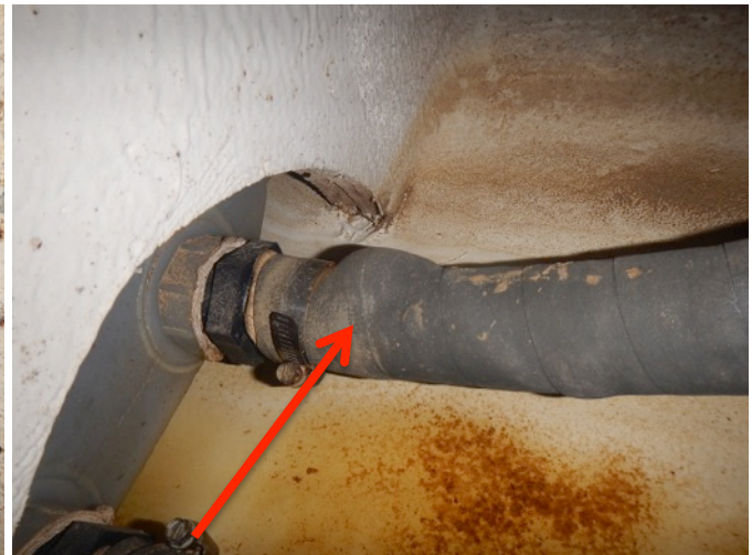
Sanitation system hoses are bulging & leaking
