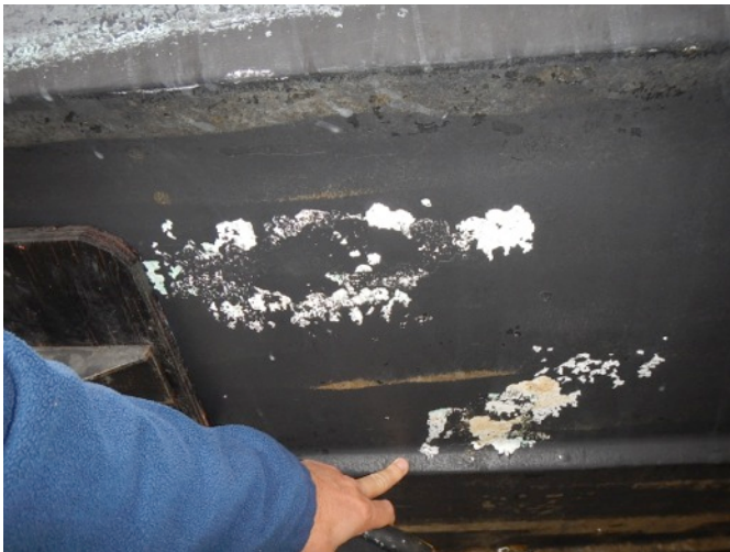
Bottom paint is deteriorating
